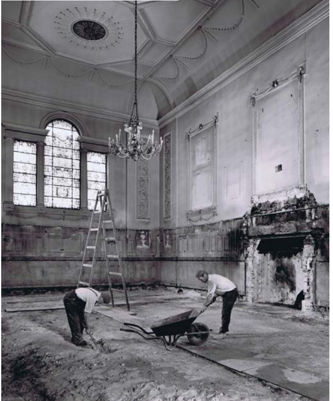
Hall during restoration 1966 – “Works to install under floor heating in 1966”
